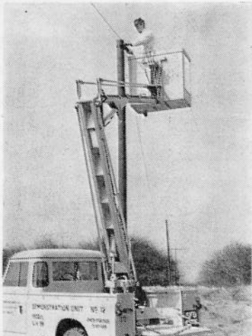
Hydraulic platform gives workman a lift.
