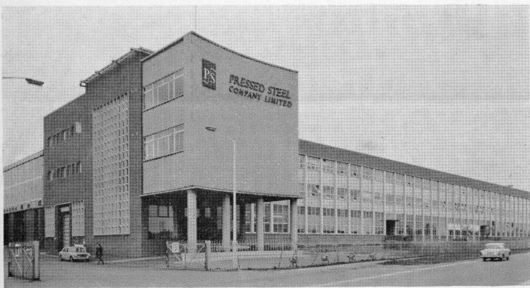
One of the six major factories of Pressed Steel Fisher—their modern and highly automated plant at Swindon
