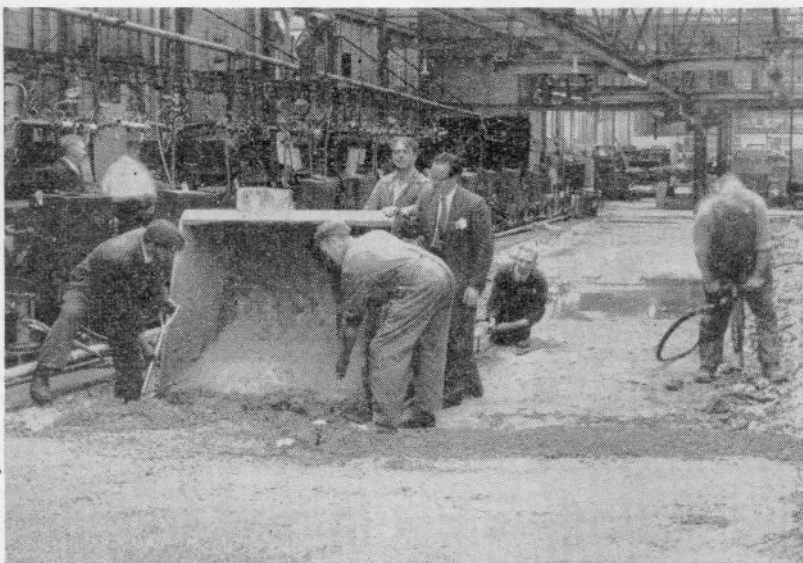
Laying new flooring in the engine test section at Tyseley.
